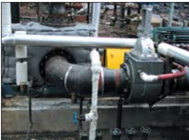
L3 re-engineered pumps replaced twin screw pumps in asphalt flux and asphalt transfer applications
