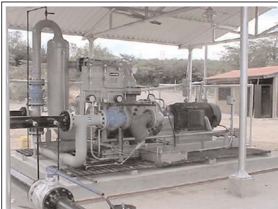
In the 25-year-old San Francisco Field in Colombia, multiphase pumps were installed in remote parts of the field, where wells at lower elevations could no longer flow back to the processing facility, located at the highest point of elevation. Not only did the low-flowing wells come back onto production after installing the multiphase pumps, but the lower pressure on the wellheads also resulted in a significant increase in oil and gas production.
