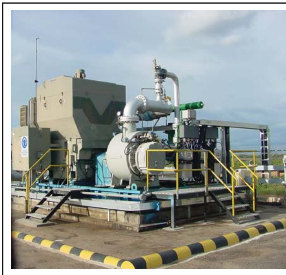
By controlling pressures, multiphase pumping enhances reservoir flow and increases hydrocarbon production and recovery while mitigating pressure-related problems from the well bore to the gathering system. Courtesy of Texas A&M Multiphase Research Group.
