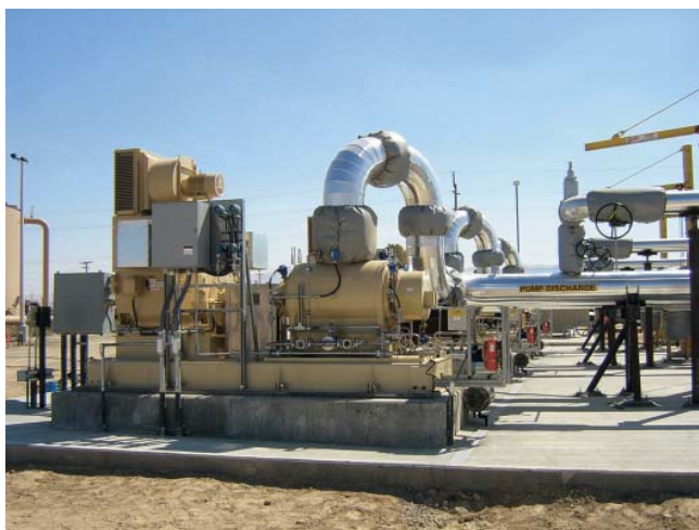
Multiphase pumps in boosting service
