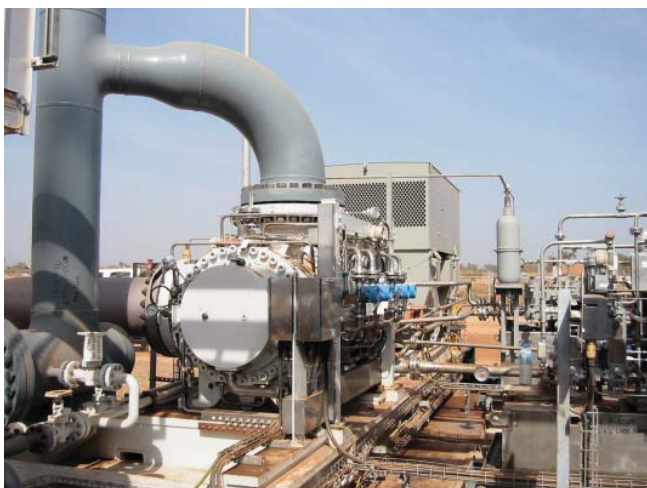
Multiphase pumps in remote site boosting service
