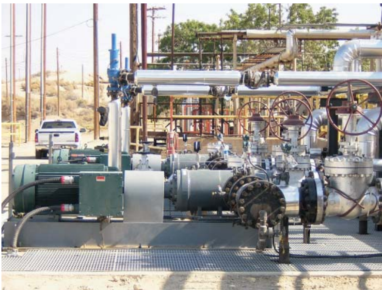
Three screw pumps in pipeline service
