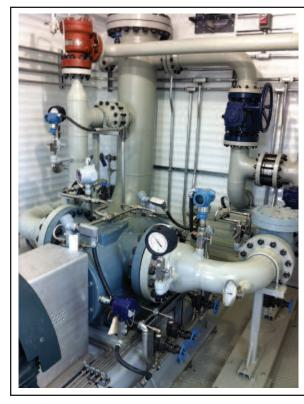
With advanced multiphase pumps, Leistritz Corp. says operators can transport oil, gas and liquids to a central location for processing without separate flowlines, separators, heat treaters, tanks, flares or stock pumps and compressors. The pumps are being used in oiland liquid-rich shales, ultradeep water, and steam-assisted production.
