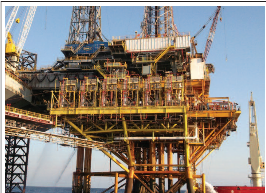
It is not uncommon for operators to run several pumps in parallel to control both the number of pumps in operation and their individual speeds so they can adjust to the number of wells flowing to a platform or pad.
