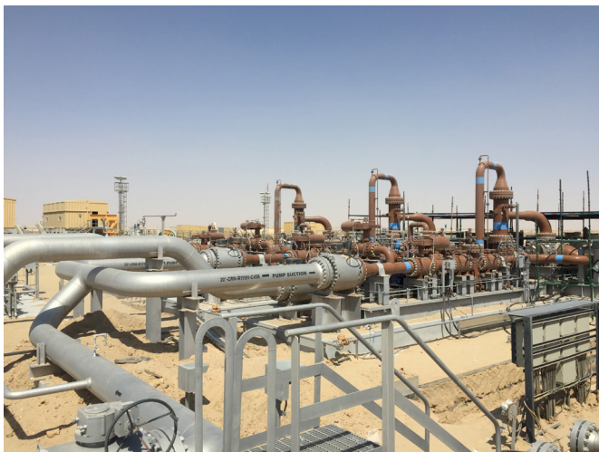
Figure 2. Multiphase gathering pump station.
